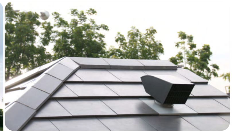
Example of a passive ventilation system, which cools the attics with natural wind at the Noble Gable Watcharapol Project
