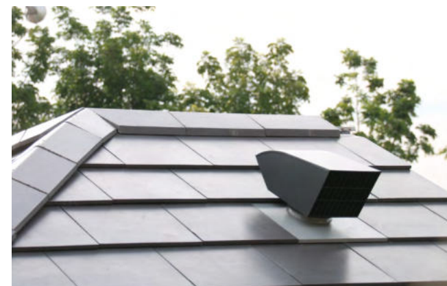
Example of a Passive Ventilation System, which Cools the Attics with Natural Wind at the Noble Gable Watcharapol Project
