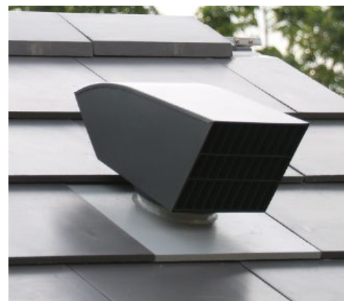
Passive Ventilation system which removing heat from the roof by natural wind, Noble Gable Watcharapol Project
